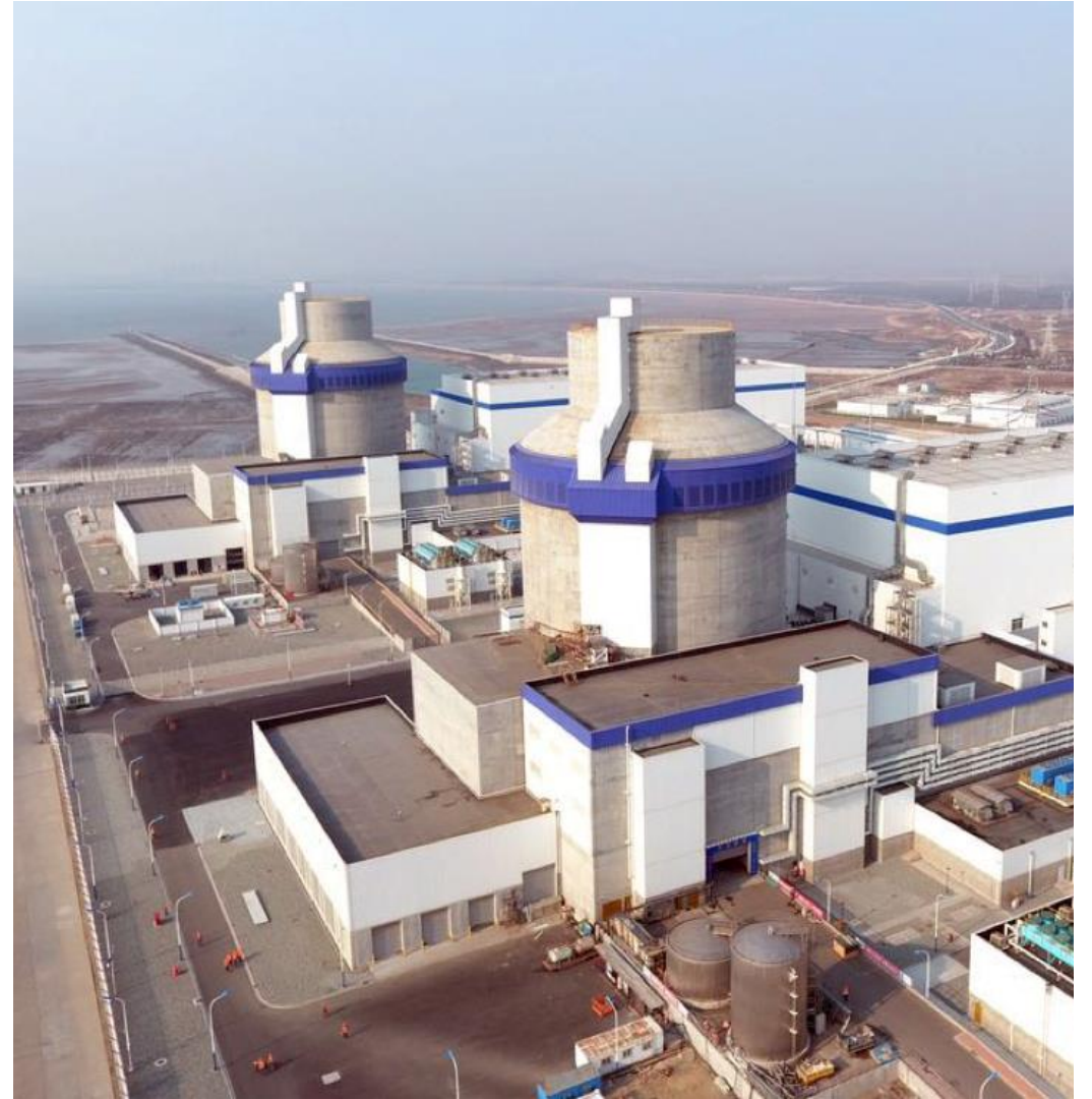
Haiyang AP1000 reactors in China with emergency cooling water tanks on top
