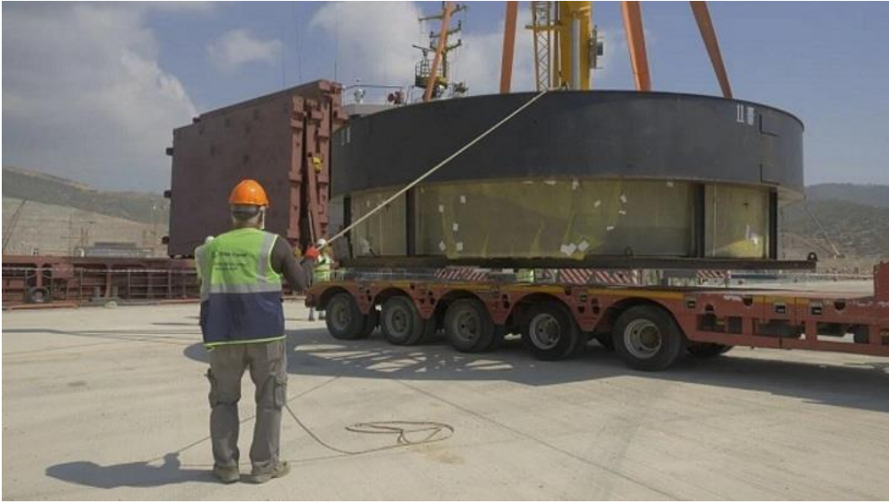
Core melt trap for VVER1200 Akkuyu, Turkey This sits under the reactor pressure vessel
